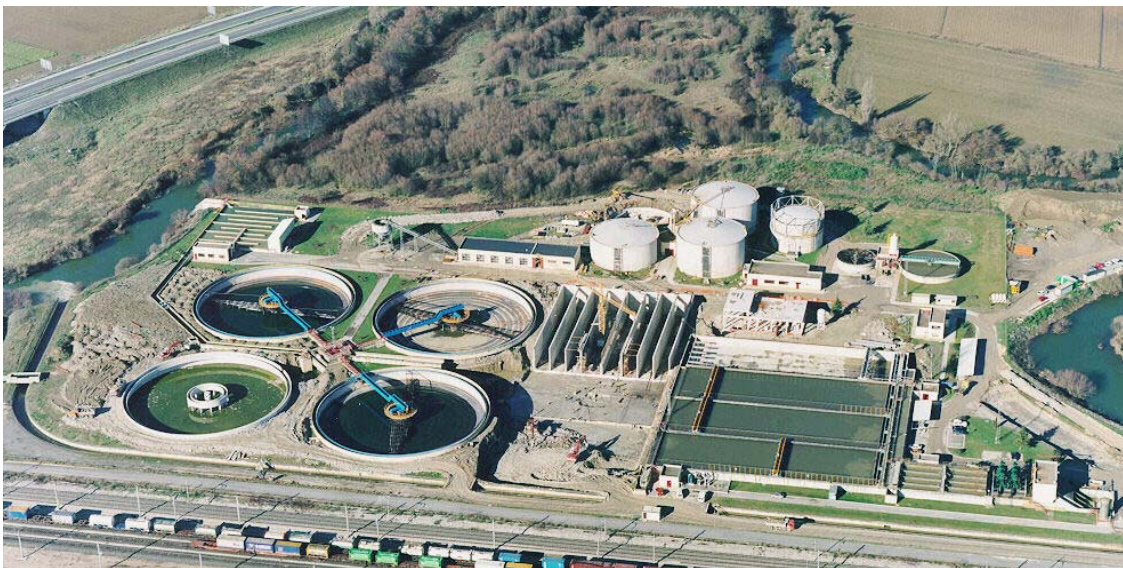
Fig. 20 Wastewater Treatment Plant of Crispijana, Spain. (Courtesy of AMVISA).
